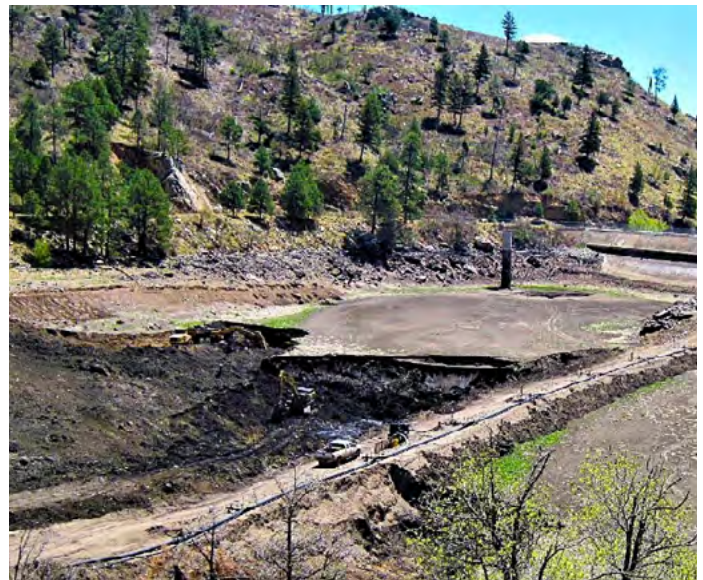
Figure 3 Bonito Dam Sediment Removal in Progress
