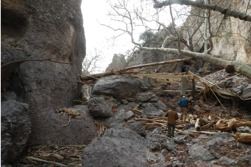
Figure 37 - Flood damage to the Catwalk, a popular tourist destination near Glenwood, NM.
