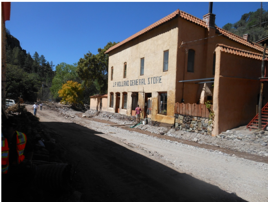
Figure 35 - High water mark on the general store, Mogollon, NM.
