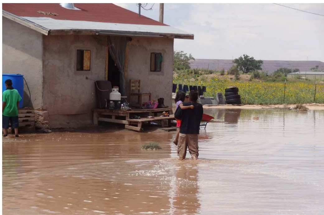
Figure 33 - Flood damage to a home in Chinle, Navajo Nation, Arizona (courtesy of Rose Whitehair).
