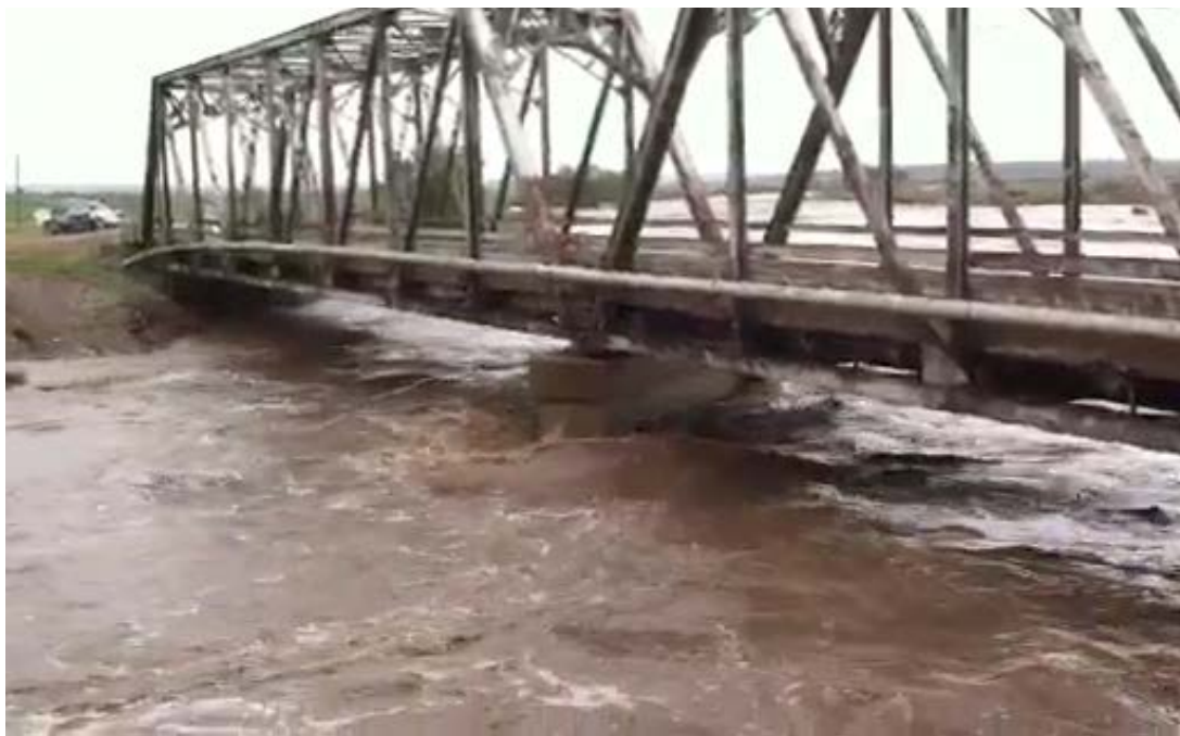
Figure 6: Rio Felix at Old Highway Bridge near Hagerman, NM (08394500), September 12, 2013. (Photograph by A. McGlone.)
